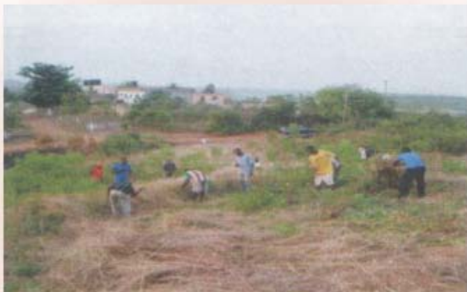
LAND BEING CLEARED FOR BUILDING
