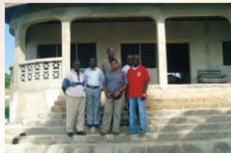
PASTORAL TEAM Standing in front of Bible School and Mission Guest House building under construction. 85% complete.
