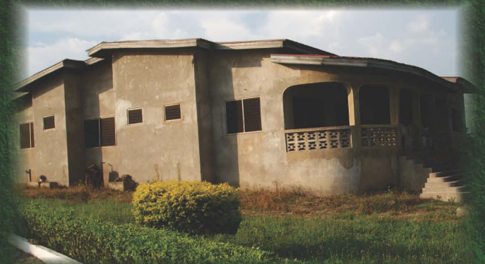
Bible School / Guest House (80% complete)
